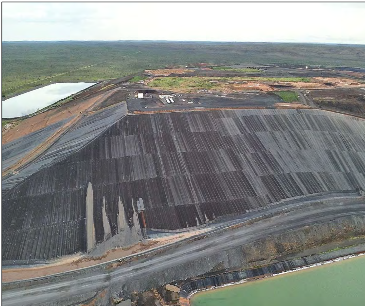
Photo 4-3: MRM drone image of NOEF BGM cover taken 16-02-25
